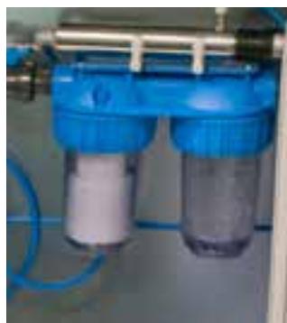
Detail of water filtering and sterilisation system
