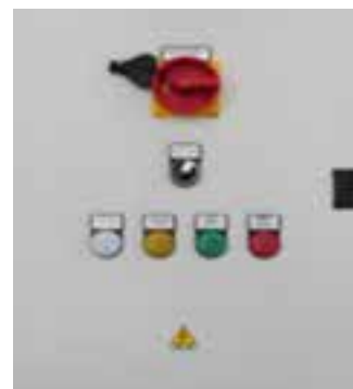
Detail of control panel
