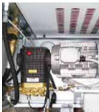
Detail of pumping system
